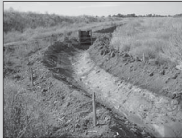
New 'V'-shaped Ditch
