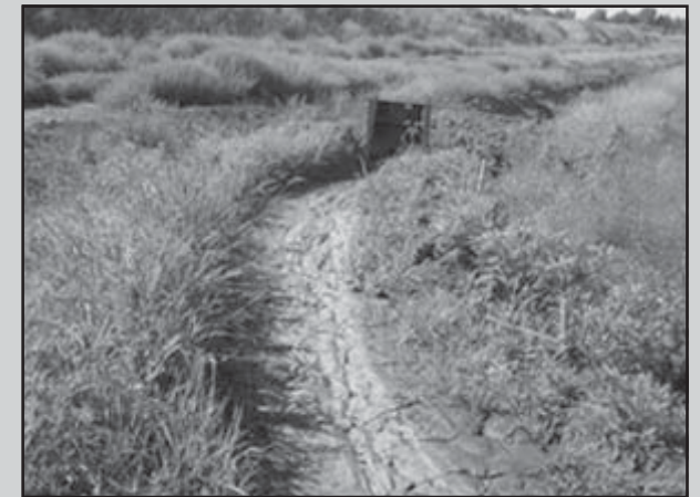
Same ditch filled with sediment
