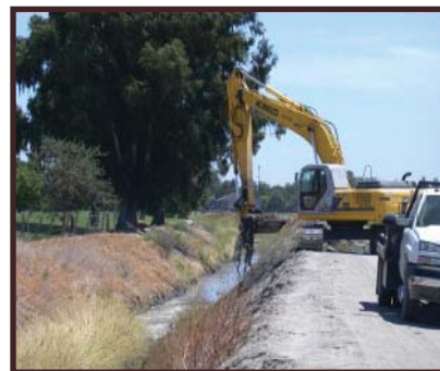
Clearing weeds from a municipal drain improves water flow and decreases mosquito habitat.
