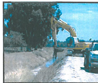
Clearing weeds from a municipal drain improves water flow and decreases mosquito habitat.
